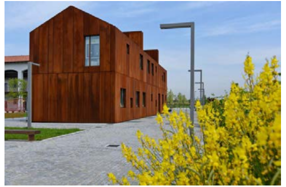
The new showroom building, inaugurated on June 9. On the ground floor are corners for each of the partners, including Allegion – CISA. On the first floor an example of an apartment.
