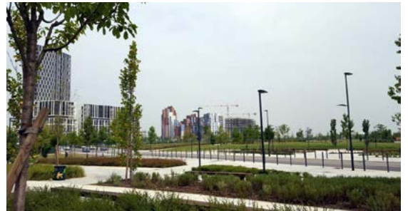
The new construction site in Milano
